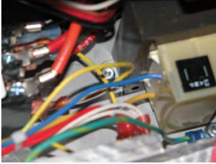
3. Use a 3/8 in. socket and extension to remove the nuts that secure the transformer to the shroud.
