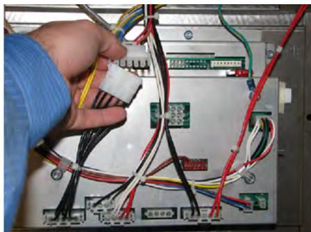
1. Lower the control board by performing the removal procedure from [5.2 Control Board Replacement, page 61](#).
