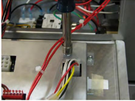
4. Use a 3/8 inch nut-driver or socket and remove the nut securing the ground wire to the control board.
